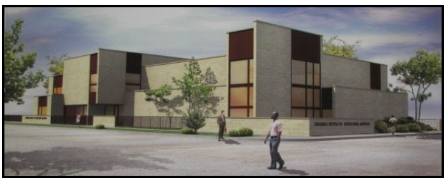
Branch 11 Headquarters: James E. Worsham Building
